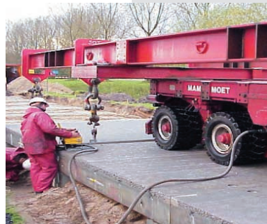
Placing of slabs on the test-section
