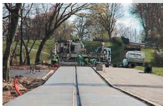
Example of internally vibrated concrete platform for pneumatic-tired tramway
