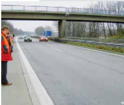
Mastic asphalt wearing course on a German highway
