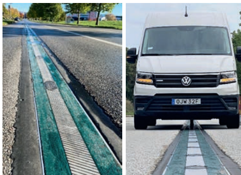
–Photos 5– Elonroad's ground conductive system (Sweden).
