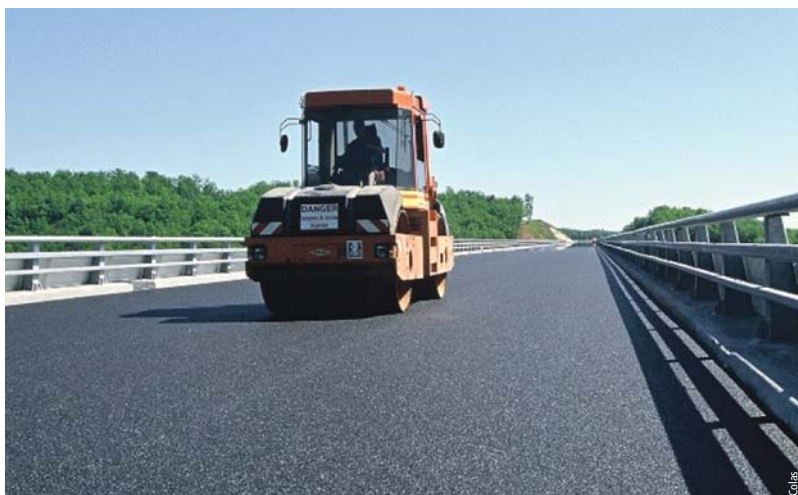
Déviation d'Angoulême, bétons bitumineux 0/6 continu Angoulême diversion, continuously-graded 0/6 asphalt concrete
