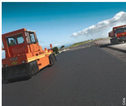
Photo 4 Atelier de compactage Compacting equipment
