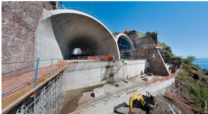
Photo 6 Tranchée couverte Saint-Paul Saint-Paul cut-and-cover tunnel
