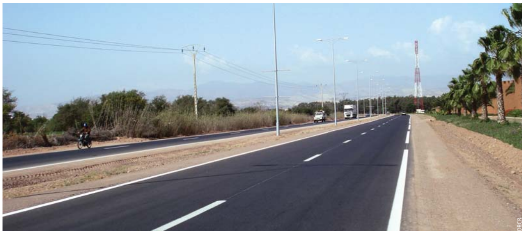
Photo 3 Voie express renforcée en BBME Express highway with high-modulus asphalt overlay
