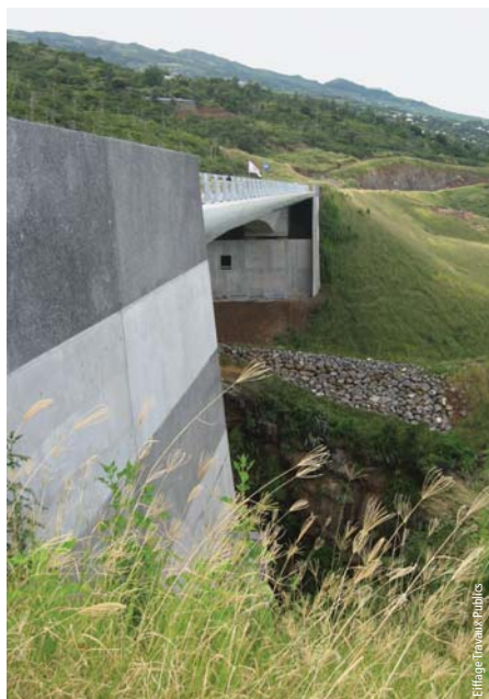
Photo 5 OANC de la Ravine Chaloupe Chaloupe Ravine, non-current engineering works (OANC)
