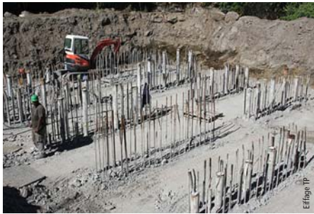
Photo 4 Injection des fondations Injection of foundations
