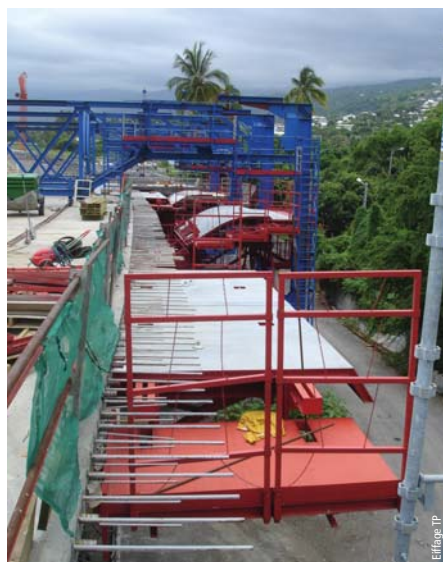
Photo 2 Equipage mobile Launching system
