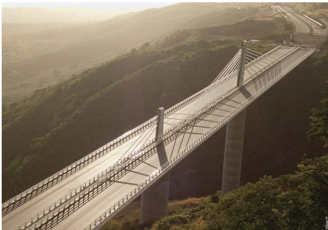
L'ouvrage terminé The completed structure
