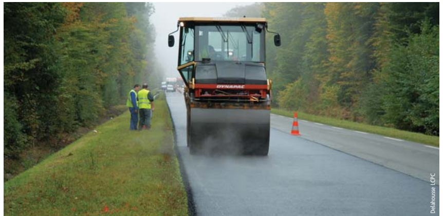
Entretien d'une RD Maintenance of a departmental (county) road
