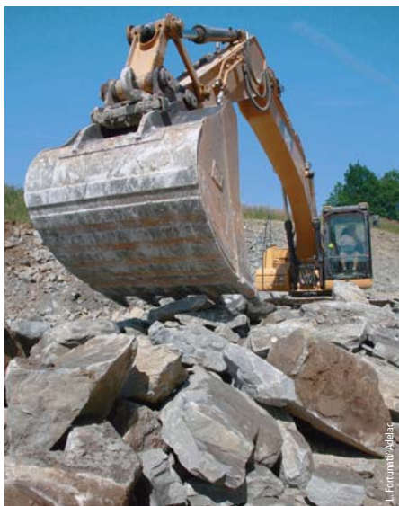
Photo 8 Echelon de pelle Fleet of excavator
