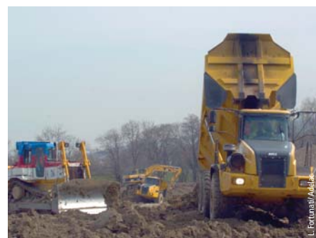
Photo 7 Bull, pelle et dumpers en action Bulldozer, shovel and dumpers in action
