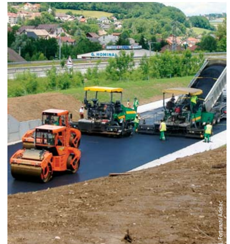
Photo 13 Application de Rugocompact, barrière de Villy-le-Pelloux Application of Rugocompact, Villy-le-Pelloux barrier
