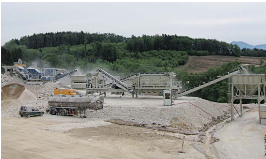
Photo 11 ICPE – Installation de concassage des aires de la Caille Facility classified for environmental protection – Crushing plant for the La Caille areas
