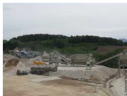
Photo 9 Installation de concassage Crushing plant
