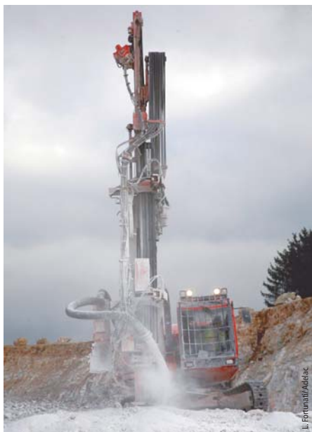
Photo 9 Foreuse Drilling machine
