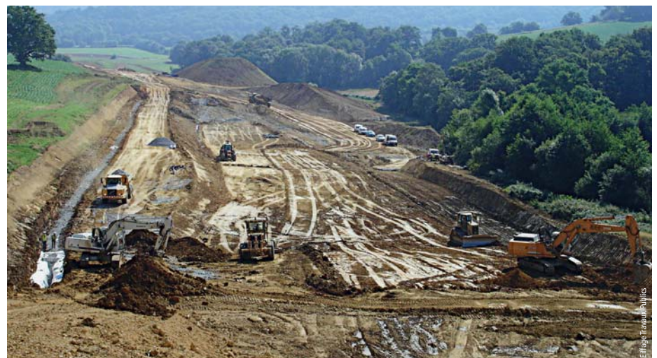
Photo 5 Remblai sur pente R123 Embankment on slope of road R123
