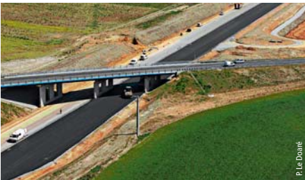
PS en dalle BP Overpass with prestressed concrete slab
