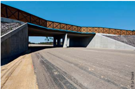
PS grande faune Big wildlife overpass
