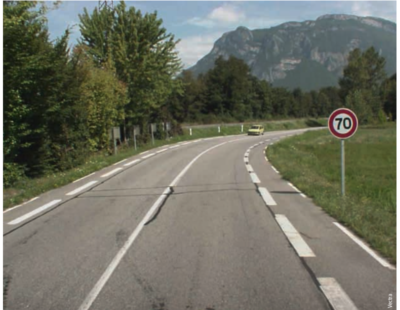
Image ASTRA simultanée au relevé de dégradations Simultaneous ASTRA image during deterioration survey
